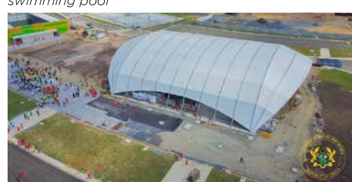
a 500-seater temporary dome
